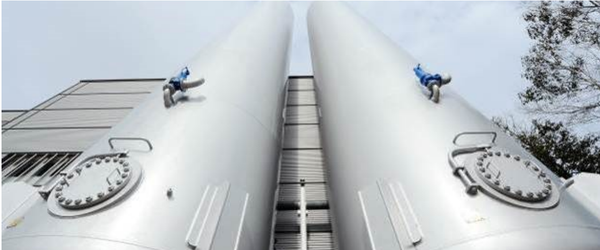
Figure 2: Reservoir pressure containers.
