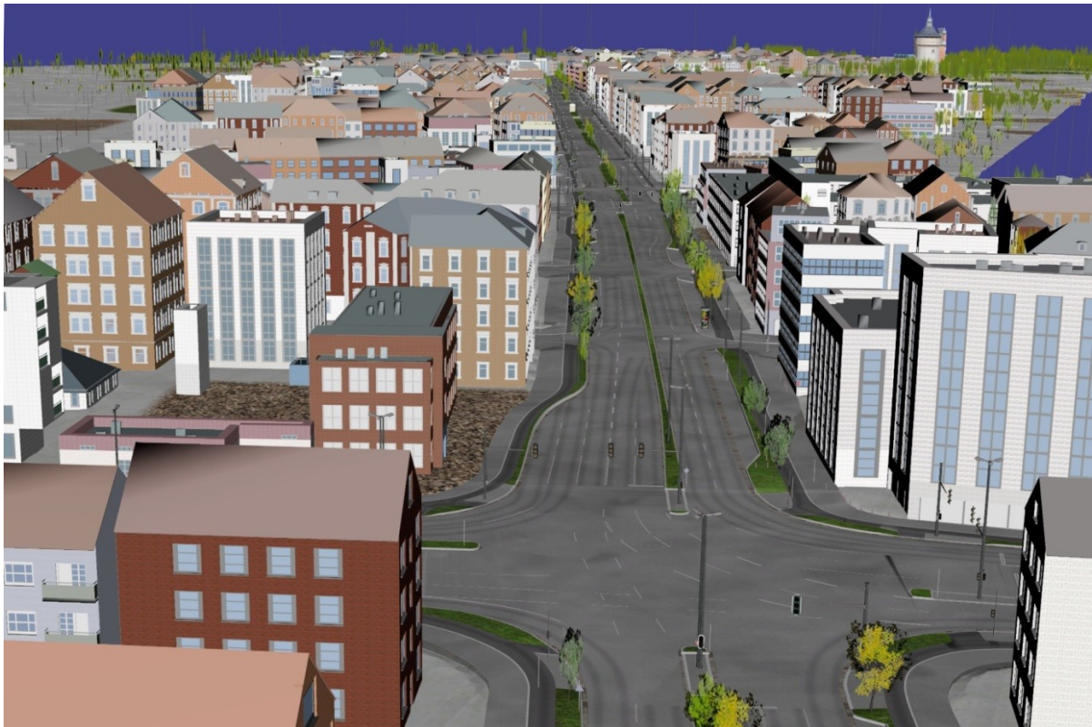
Figure 7: Braunschweiger's Hagenring towards the south.
